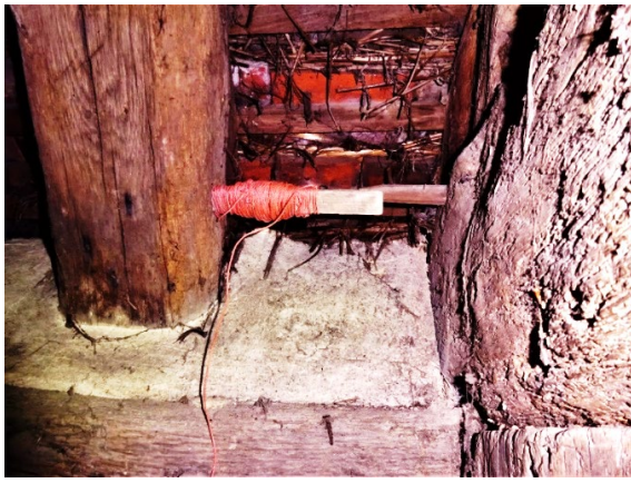
Figure 7. Rafter peg hole in line with the peg securing the tie-beam rafter on the west end of the Bayleaf tie-beam
