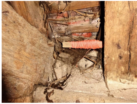
Figure 8. Rafter peg hole in line with the peg securing the tie-beam rafter on the east end of the Bayleaf tie-beam
