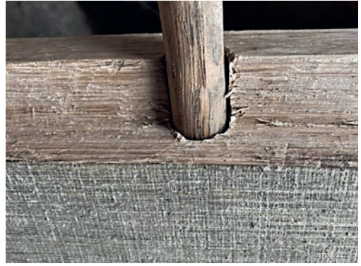
24 The peg hole is made with a shell auger to receive the location peg. Photo by E. Massey
