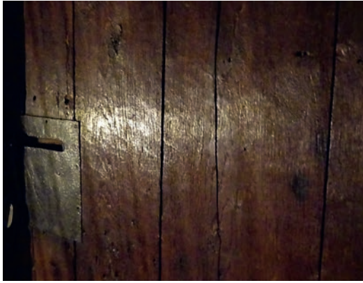
16 Tool marks seen going across the boards to remove the saw marks. Photo Paul Reed
