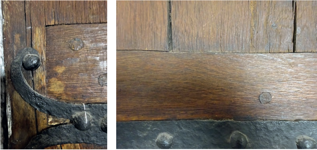
6 and 7 Details of the door, showing how neatly the ledge is let into the boards of the door. Photo Paul Reed
